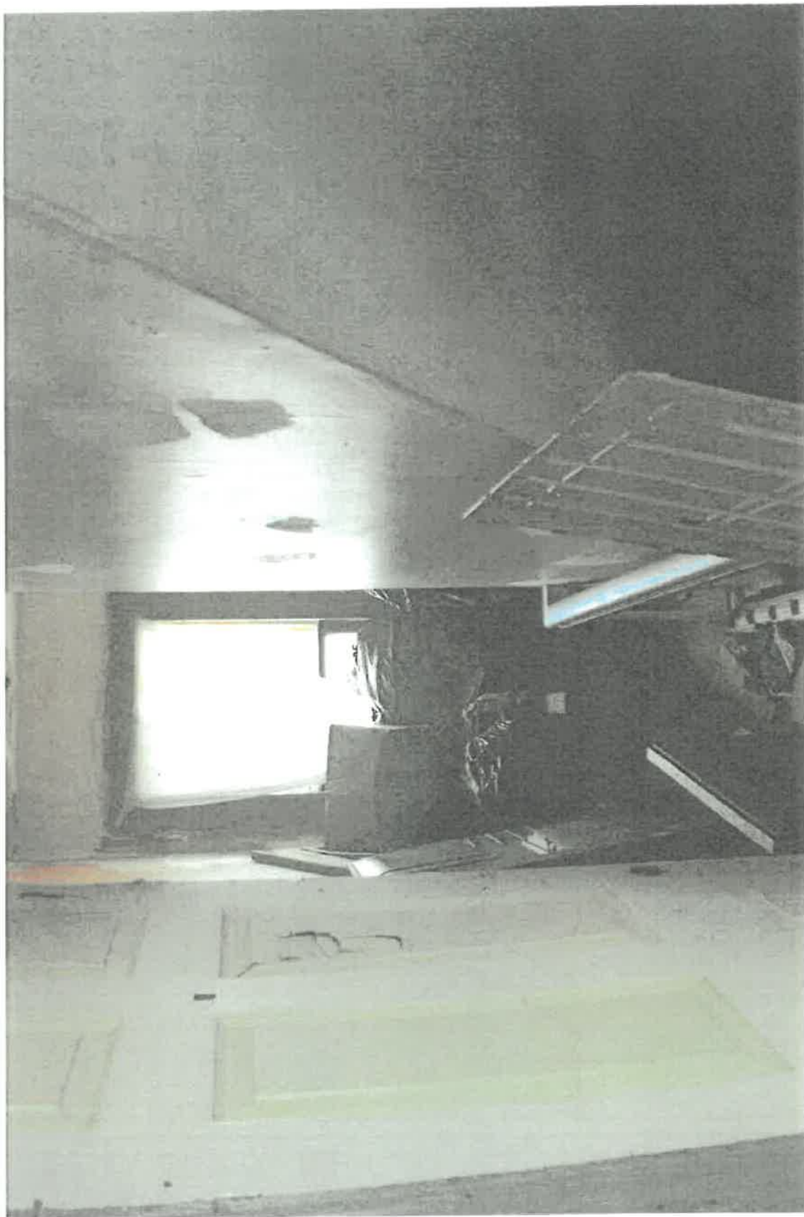
2 ND DIVISION HALLWAY FACING THE ALPHA SIDE / FRONT OF THE HOUSE
